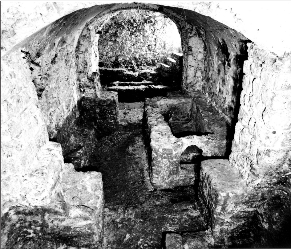
Figure 9. Gothic substructure with pre-Romanesque graves
