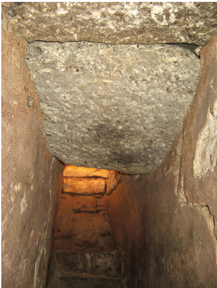
Fig. 4 Northern arm of the confessio covered with slabs of bituminous limestone
