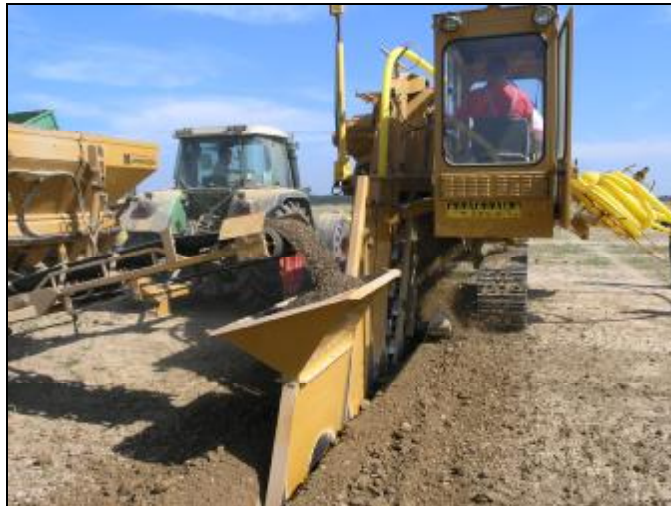
Photo 59 Drainpipe installation in a field near Popovaca
