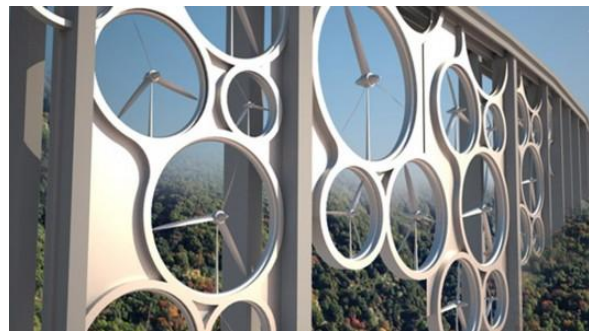
Figure 5. Horizontal wind turbine on the highway and the bridge concept, Bagnera Scilla in Italy
