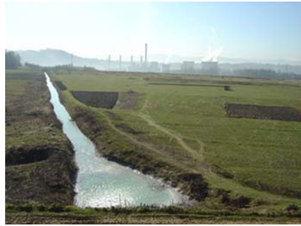
Figure 10. Release of ash transport water in Tuzla. The large particle and salt load results in the accumulation of large depositions and precipitations along the waste water canal (photos: W Fitz).
