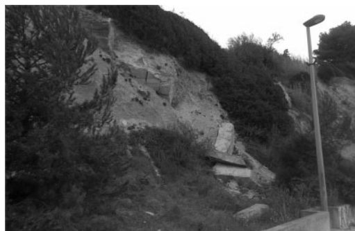
Figure 1. Example of differential weathering in flysch rock mass (Pilot site Trstenik, Split, Croatia).
