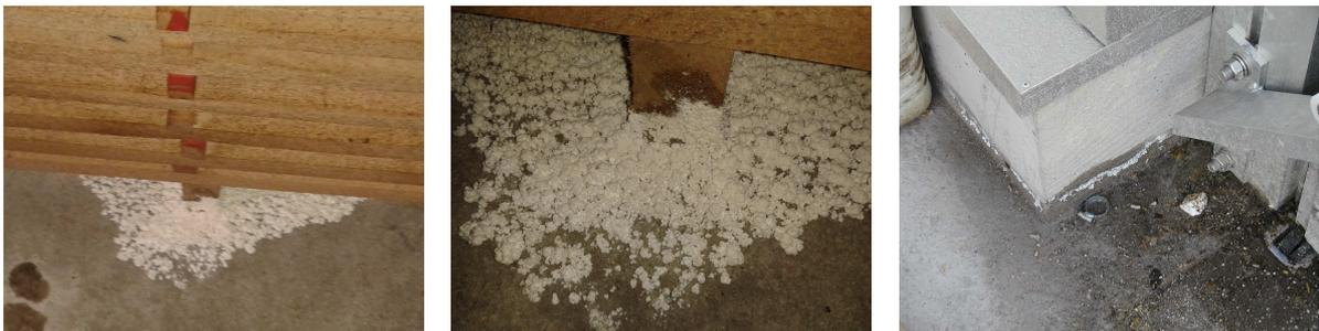
*Figure 3. Efflorescence; on wood drying kiln floor (left and middle), on the outside of reinforced concrete parapet (right) (photo: Pervan)*
