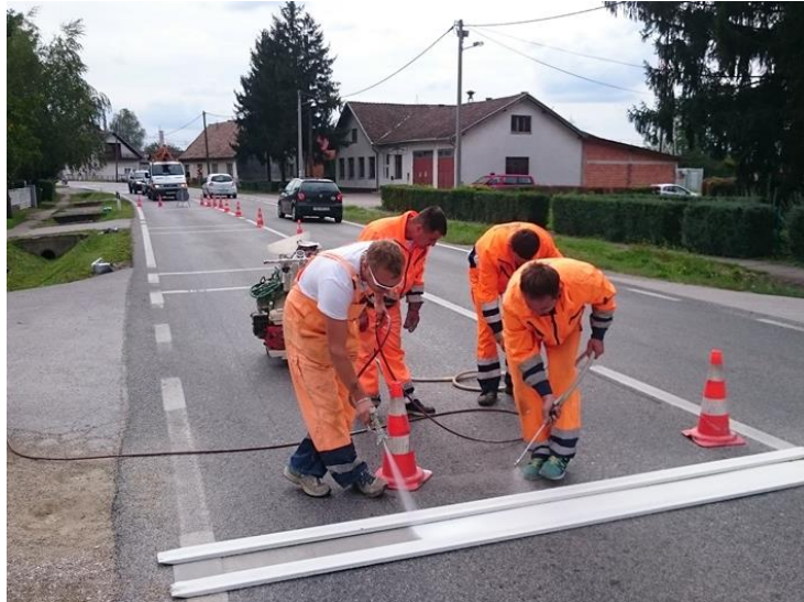
Figure 1 – Application of paint and glass beads by handheld spraying. Source: Authors.
