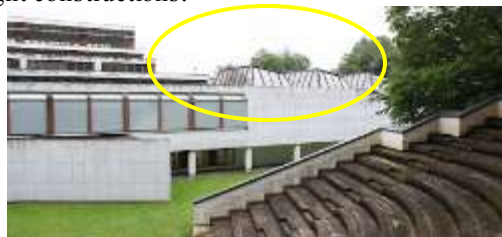
Fig. 3. Elongated skylights of the building
