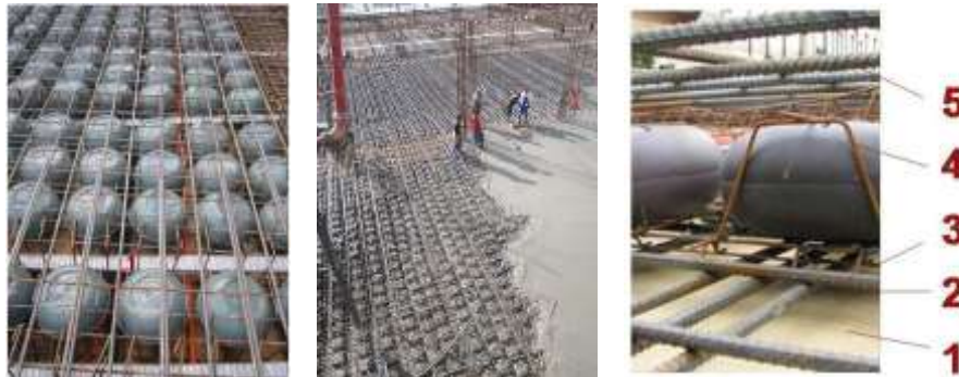
Fig 3 Realization of the slab in workplace
