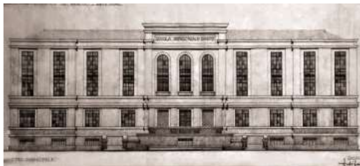
Fig. 108. Industrial School, Shkoder (Archiv of Florestano Di Fausto)
