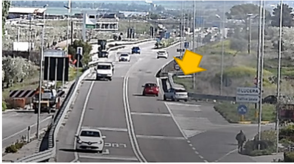
Fig. 6. Section n. 1 - Effects of the Wrong Intersection Angle
