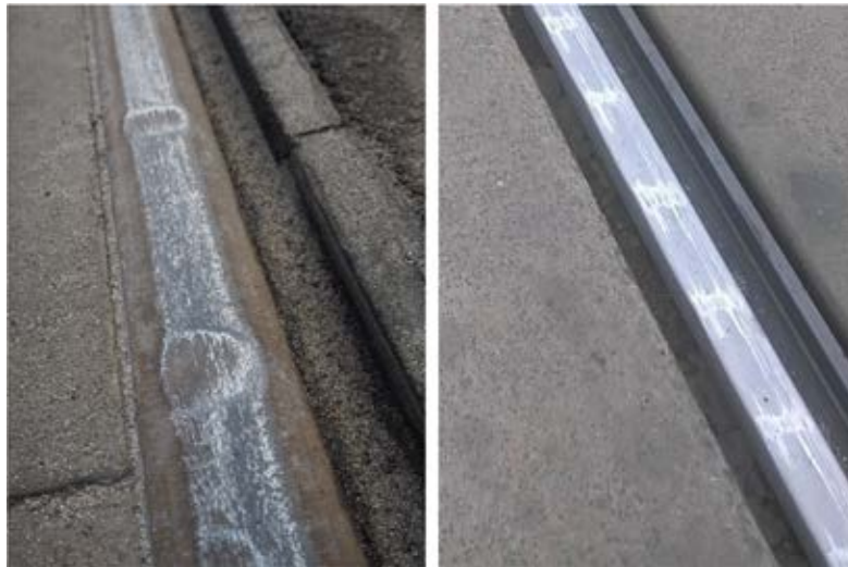
Fig. 1. Common rail defects of grooved rails
